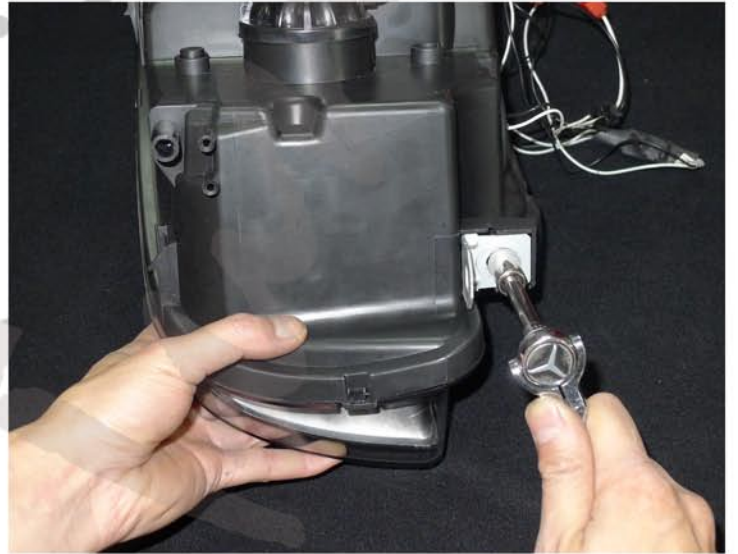
20. Place the metal bracket on the new light and tighten 10mm bolt
