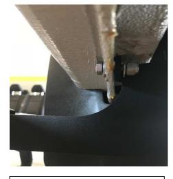
4. With step disassembled and both holes drilled, Use the 5/16 hex bolts to mount brackets as shown. Do not fully tighten.
