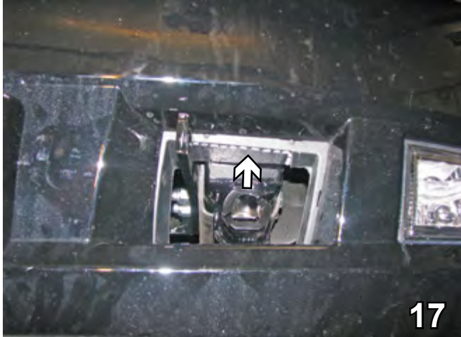
17. Cadillac Escalade: Hold the fascia in place, mark it on each side of the baseplate and cut the top of the tow hook opening so that the fascia will go back a little farther. Do this to both sides of the vehicle.
