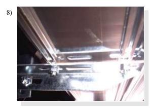
Place the board on the brackets with the bolts through the slots. Fasten with 1/4" nuts.
