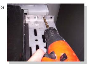
Attach FL73 to support with 5/16" bolt and nut. You will need to drill a 5/16" hole through the support for the second bolt.
