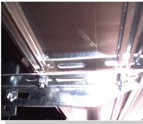
Place the board on the brackets with the bolts through the slots. Fasten with 1/4" nuts.
