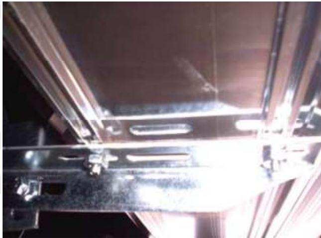
**Step 10:** Tighten all remaining nuts and bolts. Make sure every one is tight to reduce rattling.
