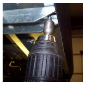
Position board up to body for best fit. Install self drilling screws through brackets into the shoulder of the steel channel on the bottom of the board.
