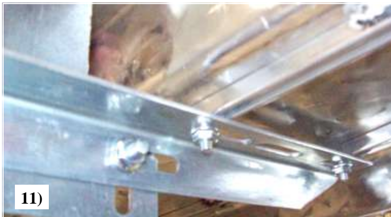
Place 1/4" nuts onto the bolts. Fig 11
