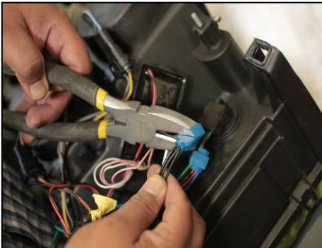
The two black wires will splice to the black wire on the same parking/turn signal socket.
