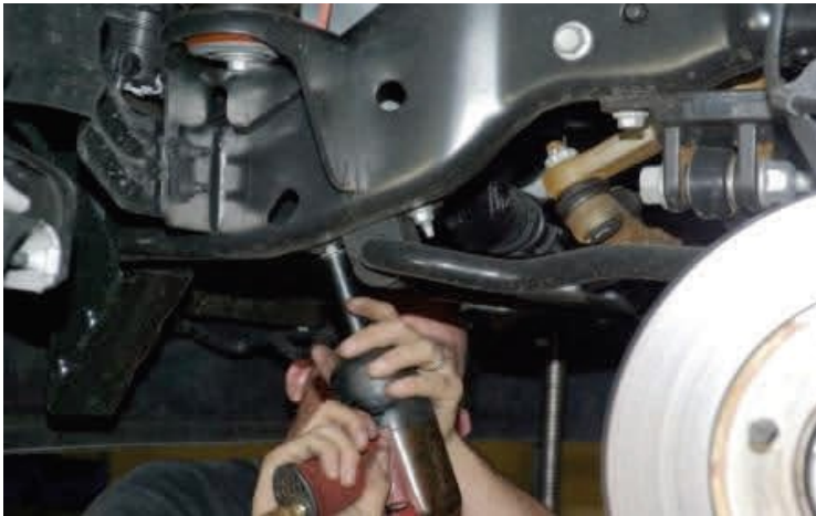
Disconnect sway bar at frame
