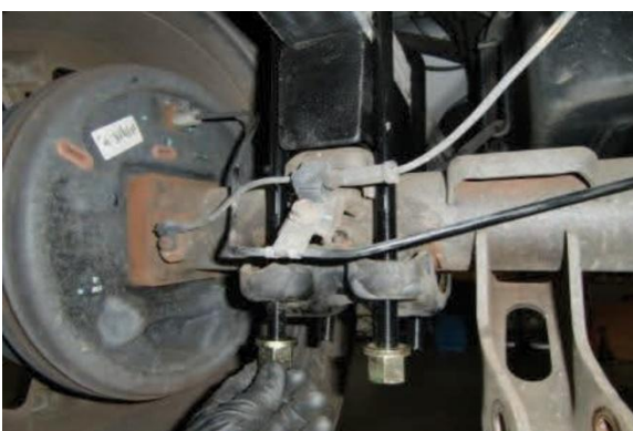
Install new, longer, U-bolts and hardware.
