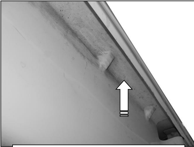
(Fig 7) Before drilling any holes through the top of the bed, check the bottom of the top edge of the bed for hardware clearance.
