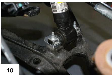
10 Image: Spacer installed.
